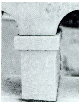
Weathering has reduced the formerly sharp edges and rounded the corners of this marble baluster. Photograph: John H. Myers.
