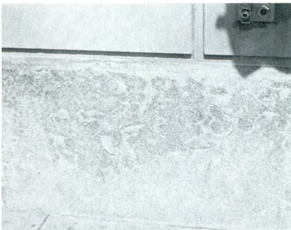
Salt fretting on granite base probably resulting from use of de-icing salts on sidewalk. Photograph: Anne E. Grimmer.
