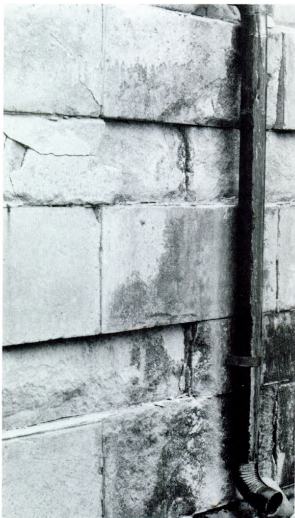
Crumbling limestone resulting primarily from excess moisture penetration. Photograph: National Park Service.
