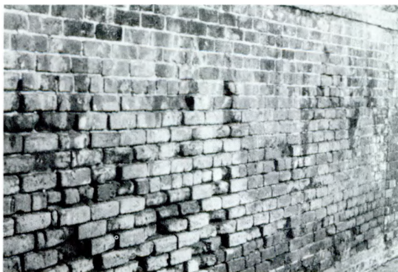
Efflorescence and spalling on brick wall. Photograph: Anne E. Grimmer.
