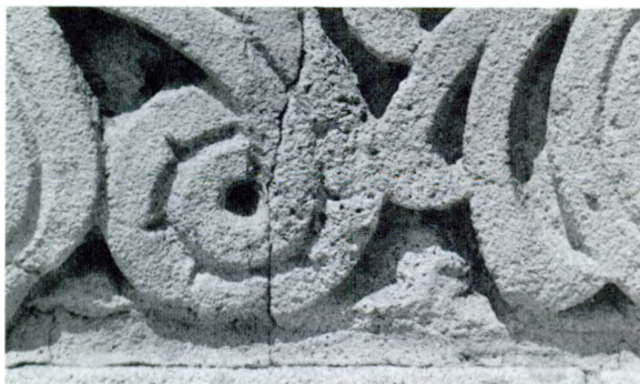
Cracking of limestone. Photograph: John H. Myers.
