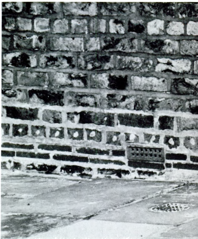
The horizontal row of white dots in the brick headers indicates that a chemical dampproof course has been injected. Photograph: Baird M. Smith, AIA.
