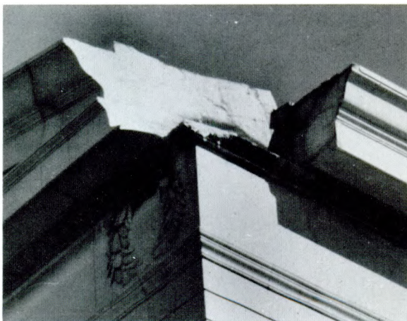
Detachment of section of marble pediment. Photograph: Walter Smalling.
