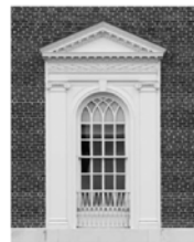
FIGURE 1 Windows are character-defining features in every historic public building. Stone quoins, Ionic pilasters and carved pediments frame multi-light, arched windows defining this Georgian revival facade. (Carol M. Highsmith Photography, Inc./GSA)
