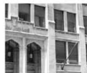
FIGURE 10 Exterior view of blast windows fabricated with custom muntin placing upper and lower panes in separate planes to simulate the appearance of double hung windows. (Mariah McGungie/GSA)
