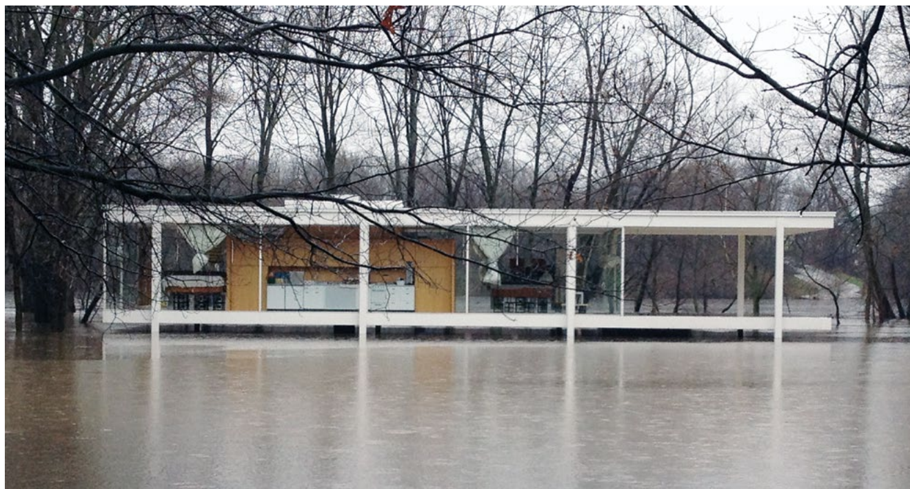
[19] The 1951 Mies van der Rohe-designed Farnsworth House, Plano, IL, was built close to the Fox River, which is increasingly prone to floods. To preserve the house in its original location, historic preservation architects and engineers continue to explore ways to protect it from the flooding, including a possible system that would lift the house above the flood waters and lower it back to the ground. Photo: Courtesy Farnsworth, A Site of the National Trust for Historic Preservation.
