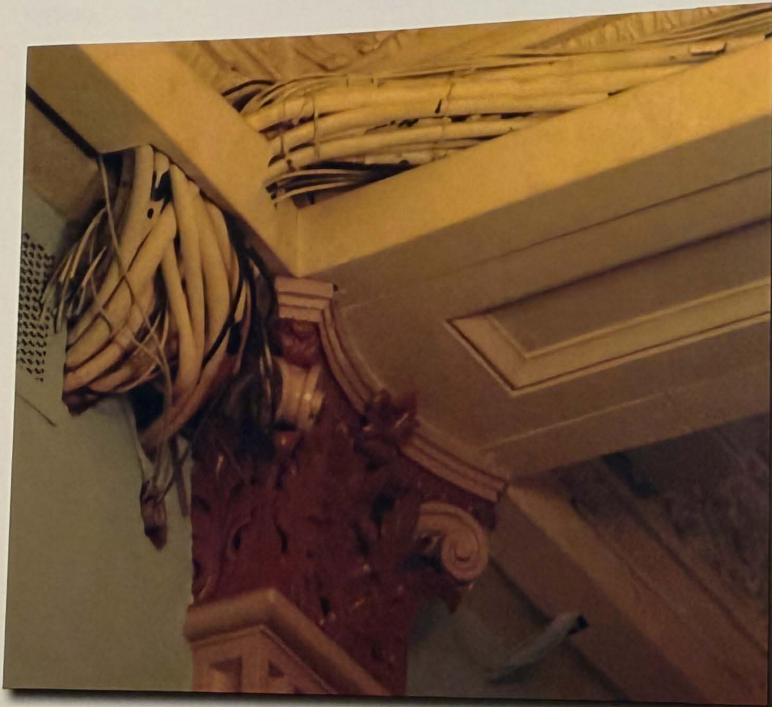
Example of original pilaster with communications lines before modernization, 2002. Pilaster is a slightly projecting column built onto a wall.
