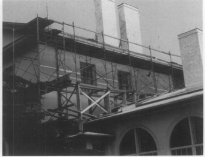
(b) Scaffolding was installed early to document existing conditions to determine extent of work.
