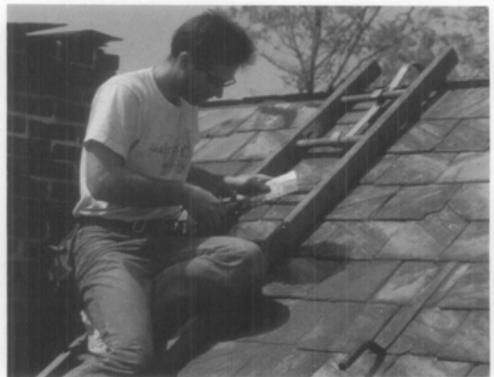
(d) A copper bib is formed to protect the newly created nail hole.
