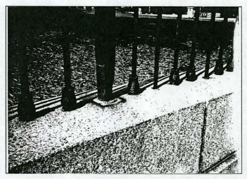
Photo 64 Deteriorated cast iron fencing along State Place. Note rusted, broken and missing elements and rust stains on granite.
