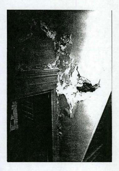
Photo 26 Note deteriorated plaster cornice adjacent to roof drain.
