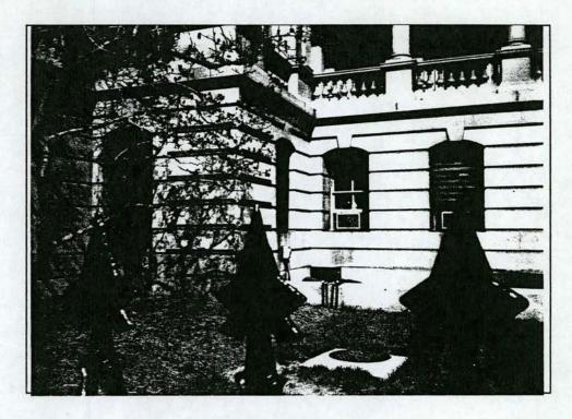
Photo 6 West elevation showing inserted window air conditioners and resulting mineral stains from condensed water from AC units.
