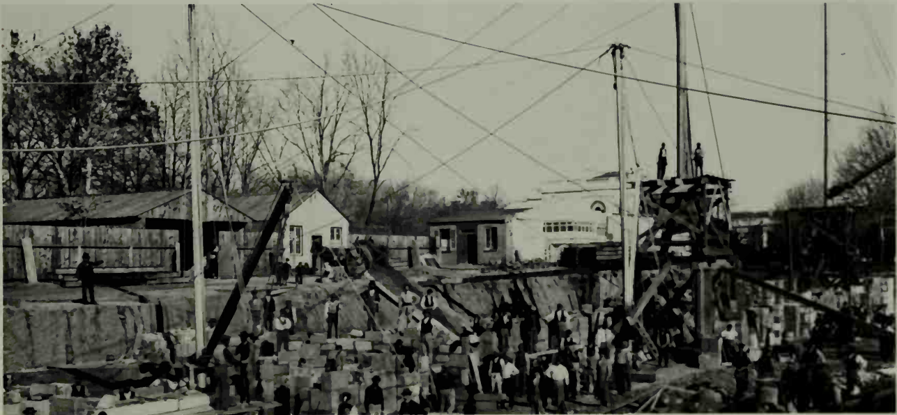
Figure 18: Construction photograph taken November 18, 1871, showing the placement of the foundation stones for the sub-basement of the State Department's south wing. The wooden derricks, each comprised of a
